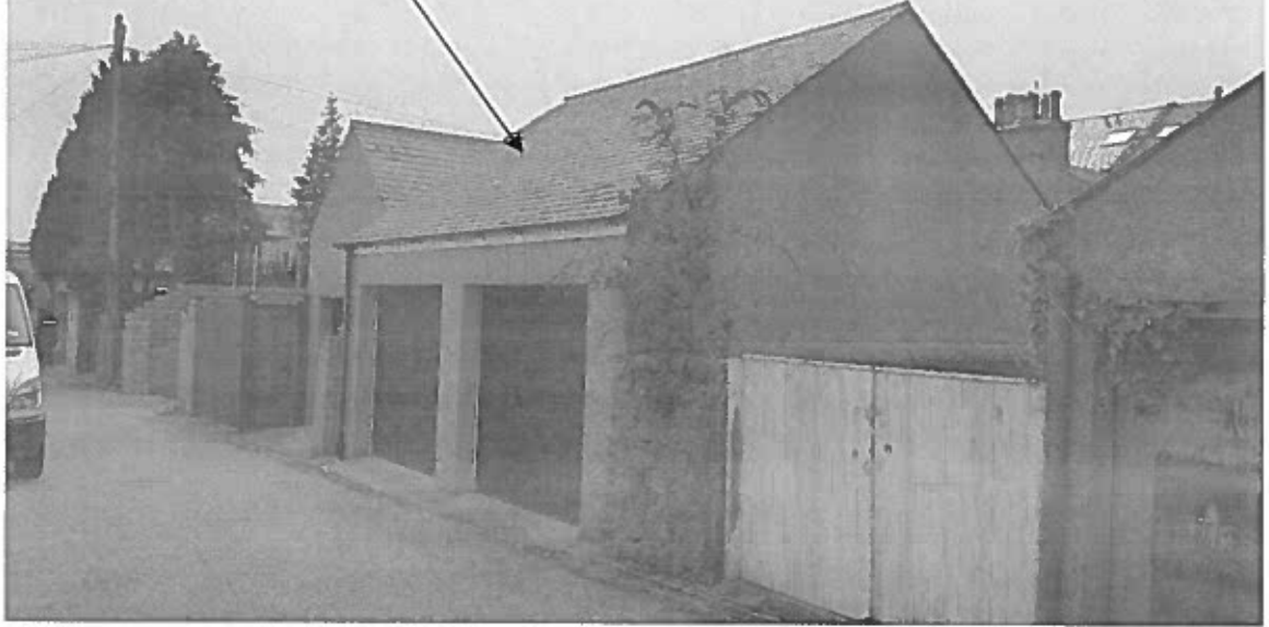
View south-east towards Desswood Place
