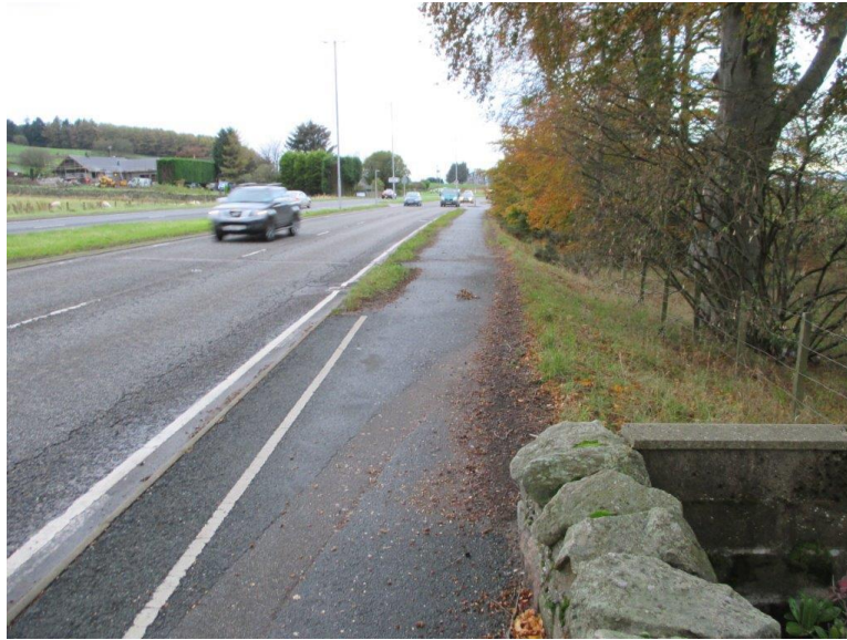
Figure 2.9 – Example of separation line.
