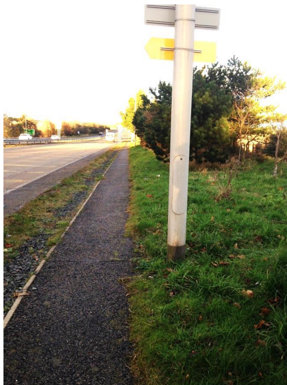
Figure 2.2 – Existing lightening columns.
