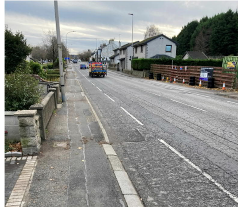
Figure 11: Stoneywood Road Advisory Cycle Lanes
