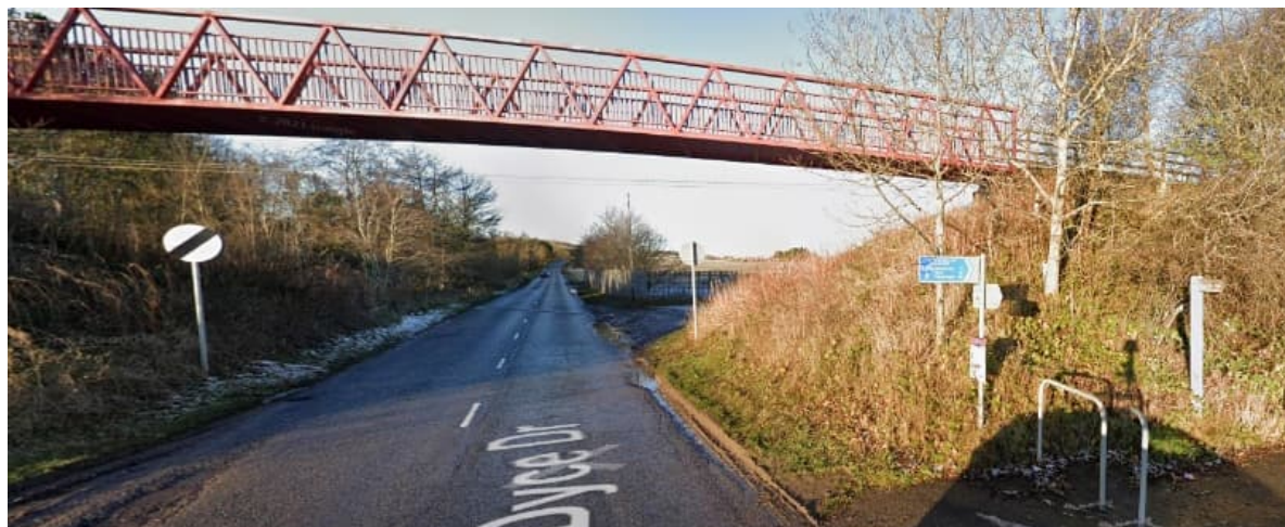
Figure 4.23: Dyce Drive Carriageway and Entrance to F&B Way (Source: Google Streetview)
