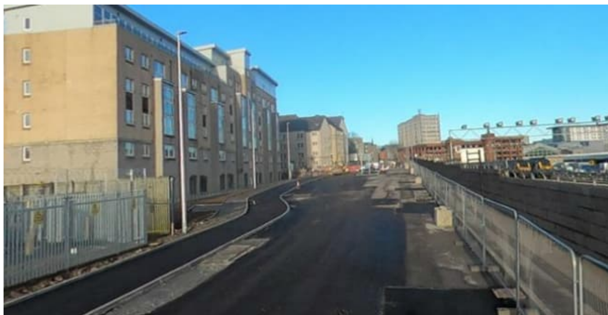
Figure 1-1: South College Street looking towards Wellington Place (January 2023)
