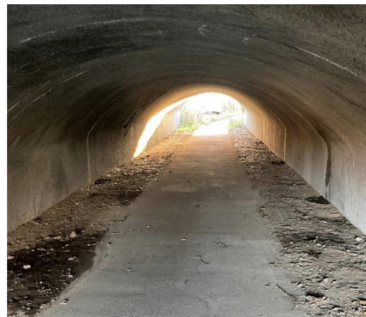
Figure 3: NCN Underpass access
