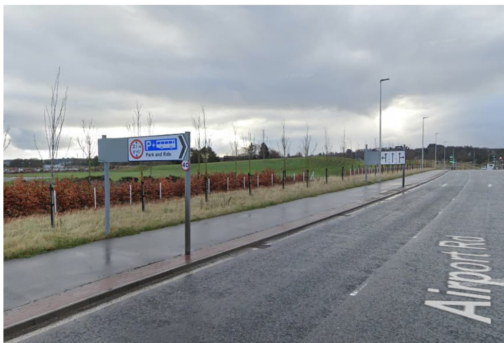
Figure 4.10: Existing Traffic Sign Mounting on Airport Road (Source: Google Streetview)
