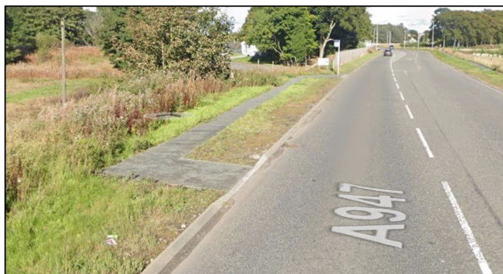
Figure 4.11: Existing Dropped Kerbs on A947 (Northbound) (Source: Google Streetview)
