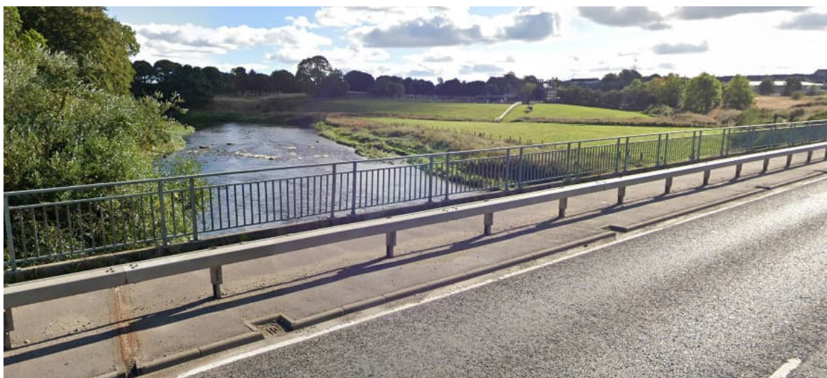
Figure 4.25: VRS Placement on Parkhill Bridge (Source: Google Streetview)
