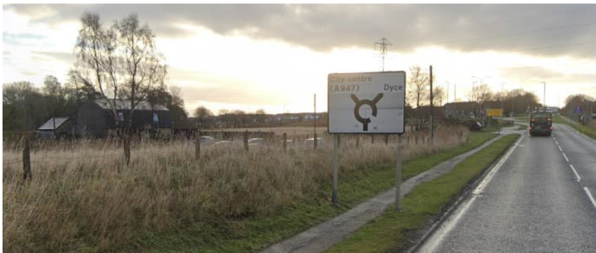
Figure 4.24: Narrow Verge with Adjacent Land Boundary (Source: Google Streetview)
