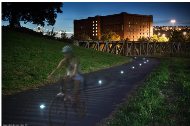
Figure 4.22: Solar Stud Lighting Example (Coe Fen Cycle Route Cambridge)
