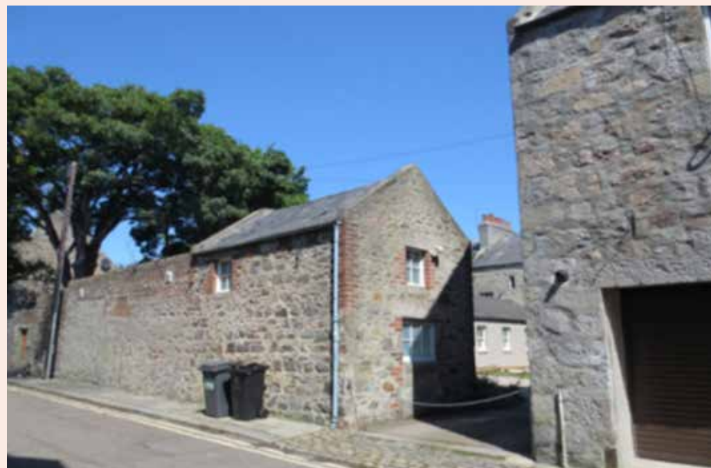
Original news building in Gordon Street now converted into a home as part of an entire feu redevelopment.
