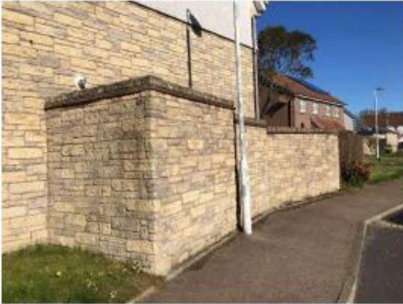
Photograph No 13 Wall at 25 Seaview Avenue
