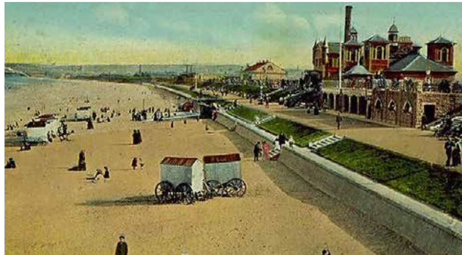
The Battery, Lifeboat Housing & Bathing Station
