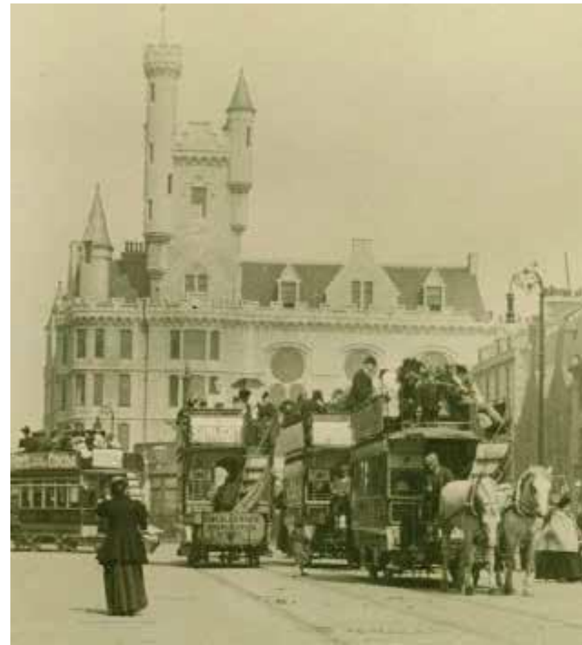
Tram Transport Hub at Castlegate
