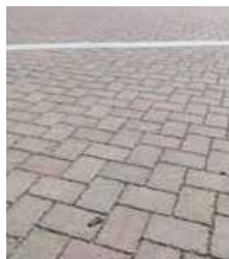
above & right Permeable Surfacing
