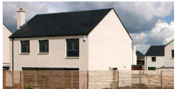
above Example image illustrating a white render finish with dark grey pitch roof
