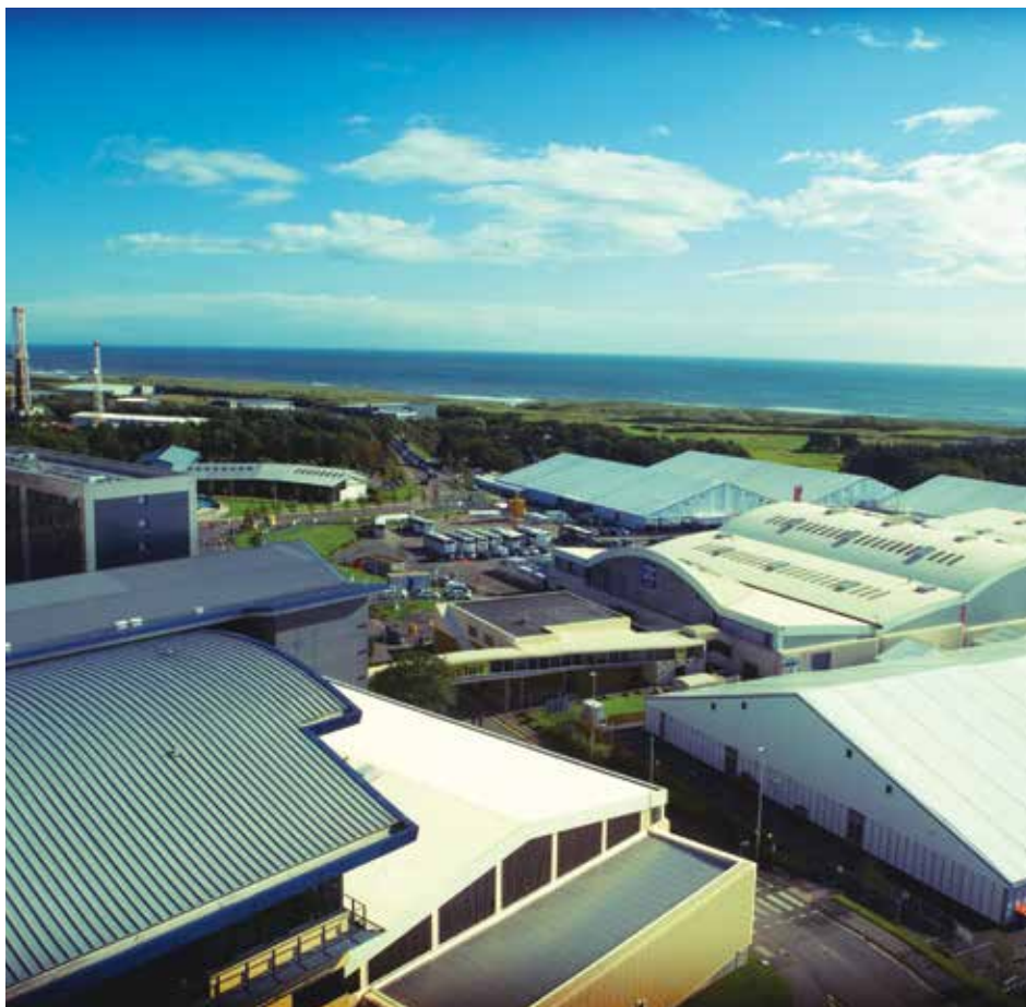
above Existing AECC at Bridge of Don
