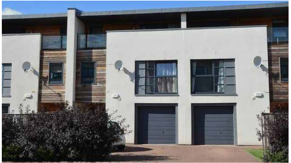
above Example image illustrating a white render facade with feature timber panels
