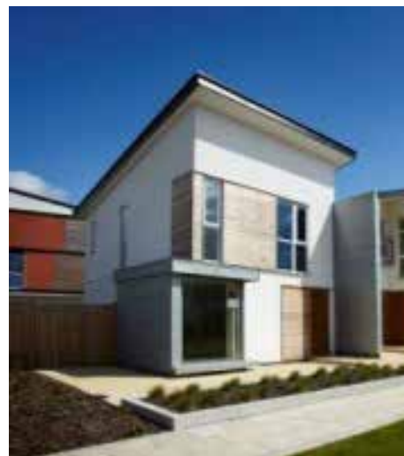
above Example images illustrating feature elements on corners & elevations to break up facade
