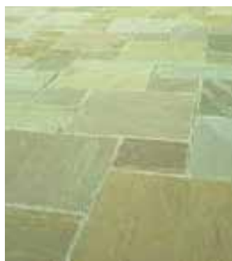
above Natural Stone Footway Surfacing
