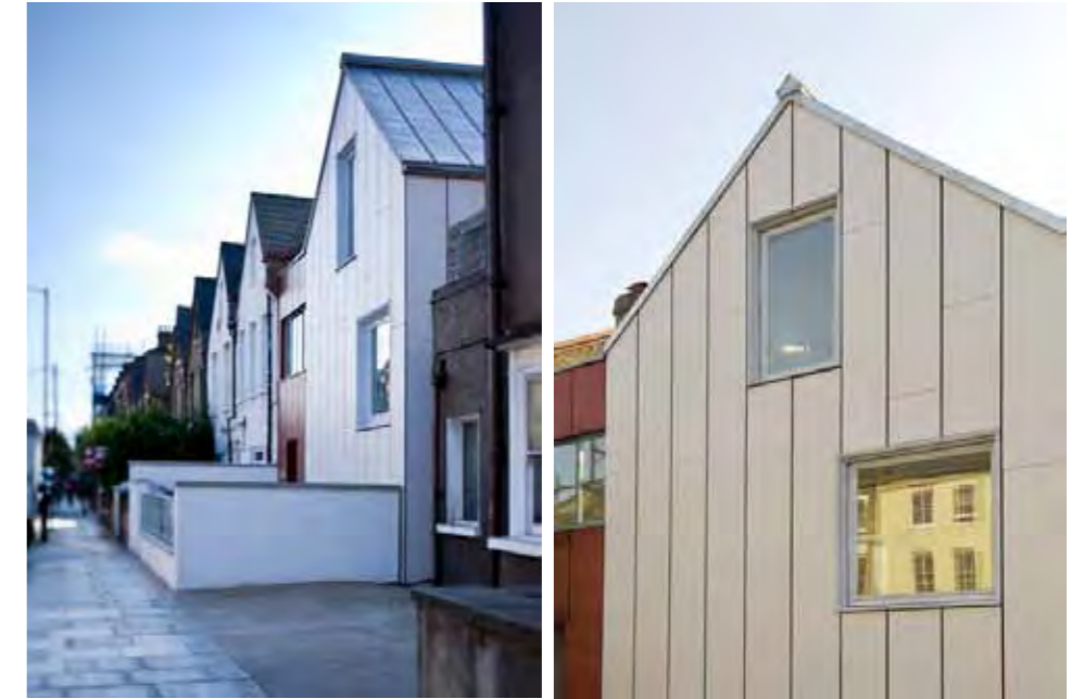
Gilliespie Road, London. Eternit Natura fibre-cement rainscreen wall cladding.
