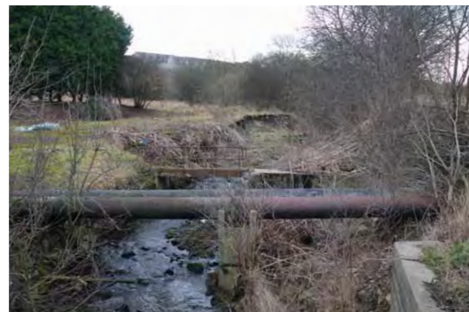
Remove redundant grilles, pipes and infrastructure
