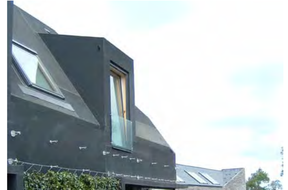
Scottish Housing Expo: Contemporary eaves dormers and rooflights.
