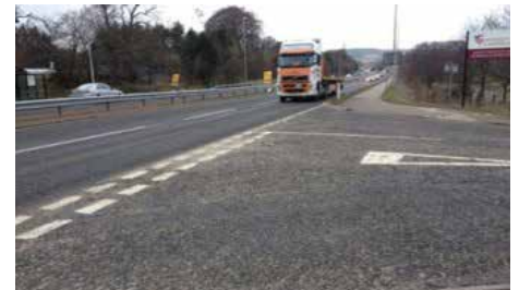
above Present A96 Access
