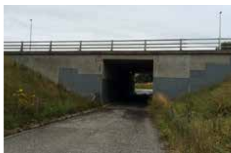
above Existing Underpass
