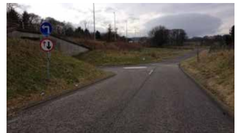
above Approach to Underpass
