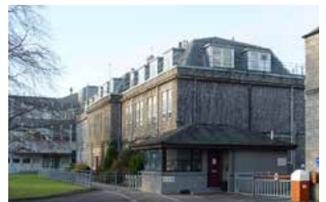
2 Boyd Orr Building
