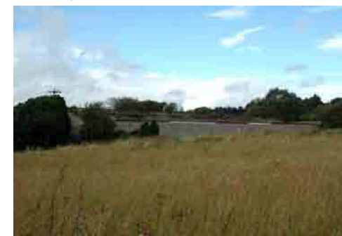
Viewpoint 17: Electricity Substation
