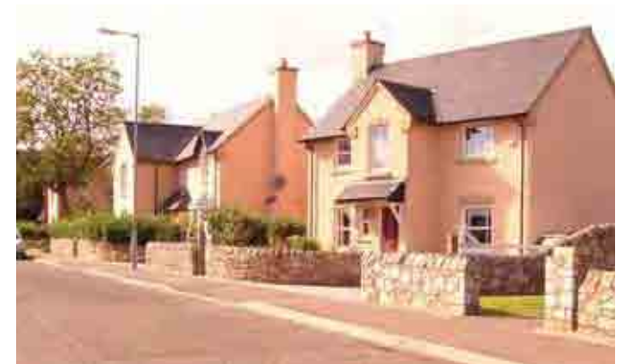
Well defined building line and plot boundaries, Scottish Borders.
