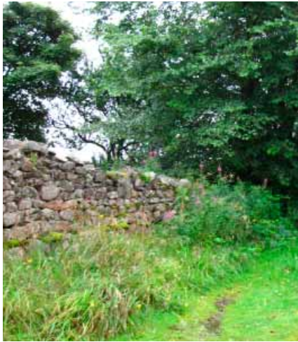
Figure 2.23 Existing stone walls on site
