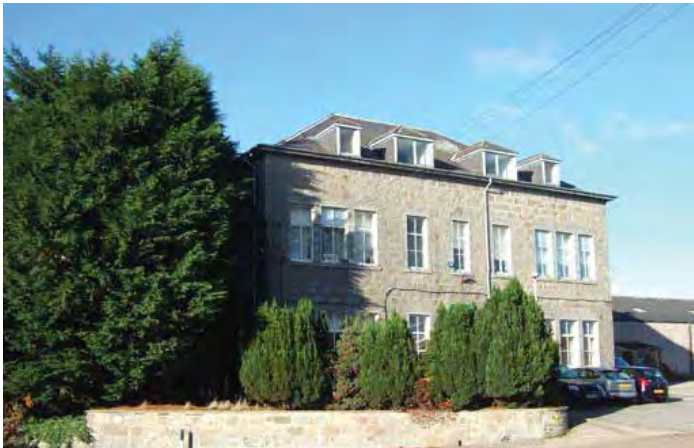
Doig Scott building - potential for retention and reuse
