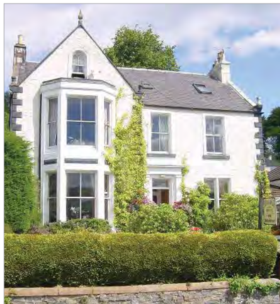
fig. 149: Detached villa overlooking street.
