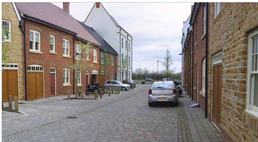
fig. 146: Shared surface street, Upton.
