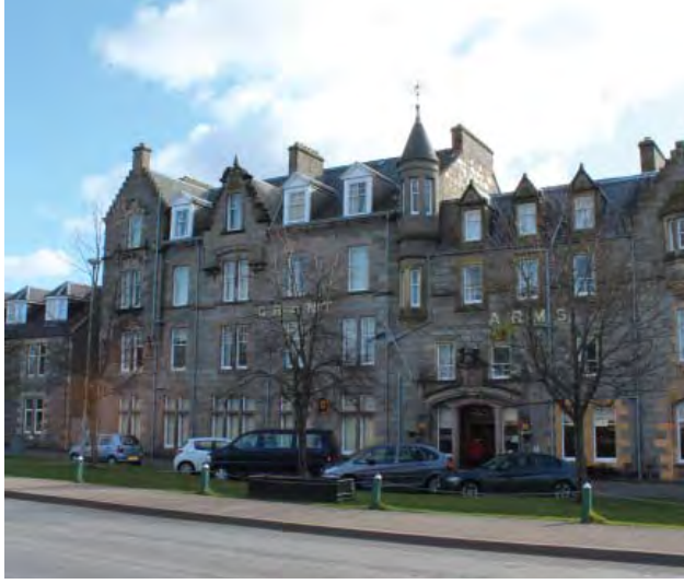
fig. 174: Built frontage to open space, Granttown on Spey
