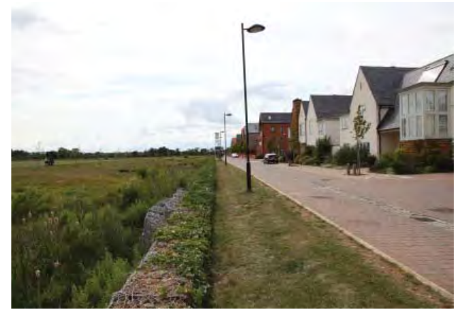
fig. 82: Buildings overlooking public space, Upton, Northampton.
