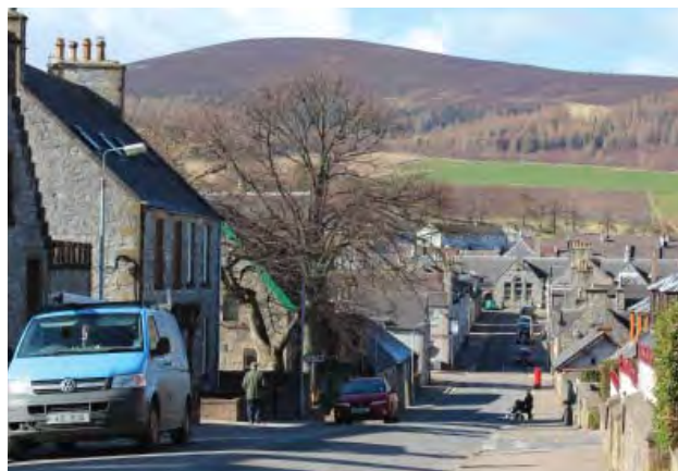
fig. 84: Landmark buildings - Dufftown
