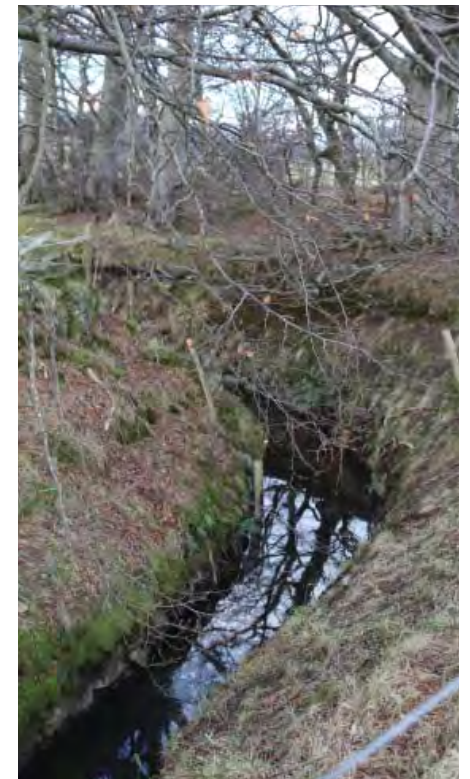
fig. 39: Existing drainage ditch adjacent Countesswells Road
