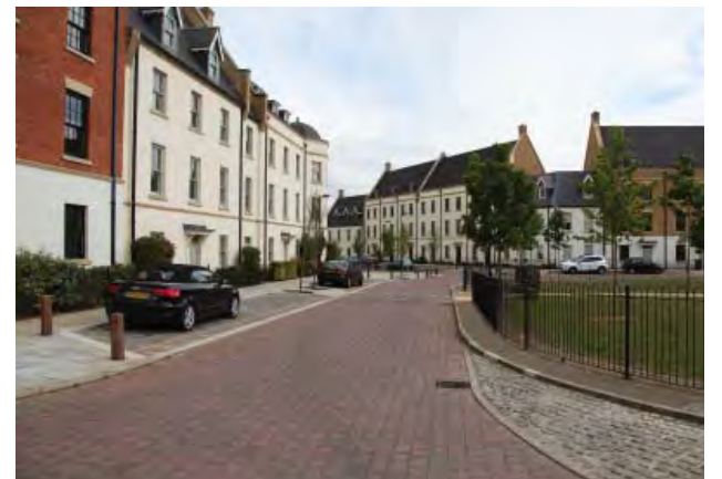
fig. 91: Residential street - Upton, Northampton
