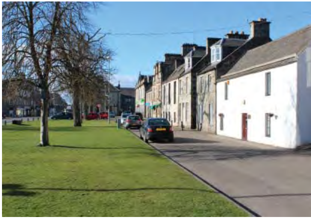
fig. 80: Buildings overlooking public space - Granttown on Spey
