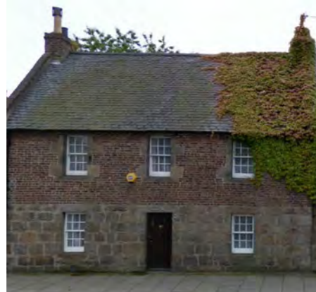
Figure 5.35: Study of Cluny's Port building proportions informing the system used in Grandhome's single family terraced houses
