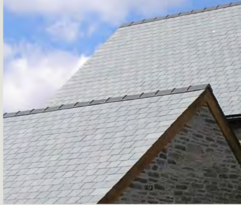
Figure 5.42: Slate roof
