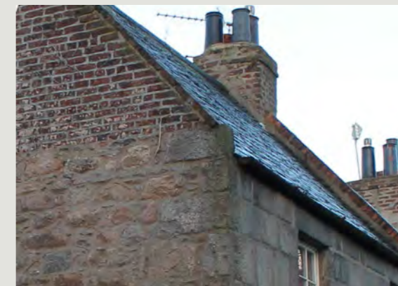
Figure 5.58: Reclaimed granite and brick gable
