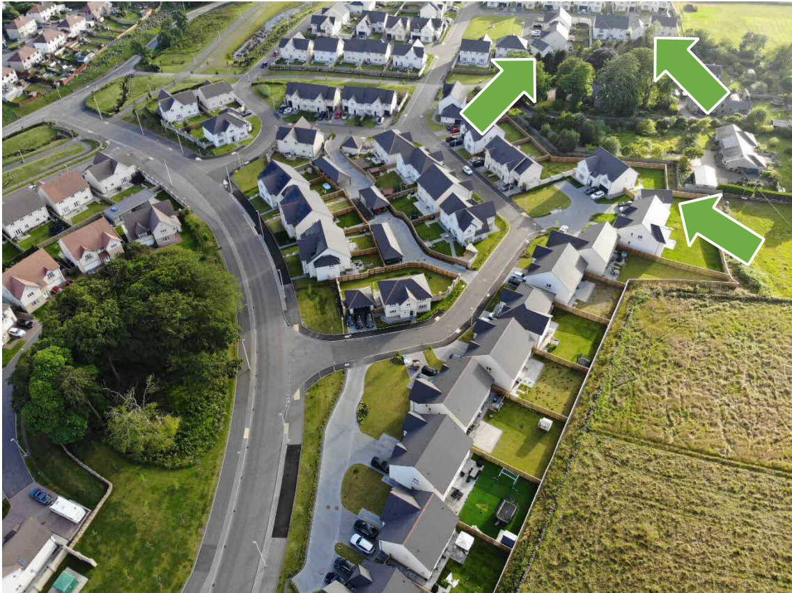
0161-01-PHOTO_003 (Aerial Photograph)
