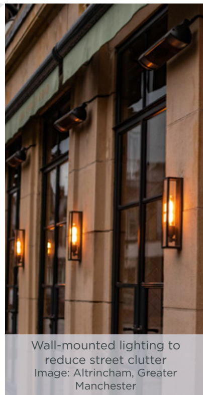
Wall-mounted lighting to reduce street clutter Image: Legend Light by Thorn Lighting.
