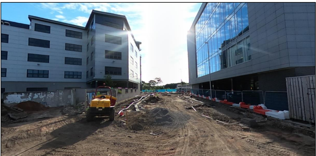
Palmerston Place looking toward North Esplanade West August 2022
