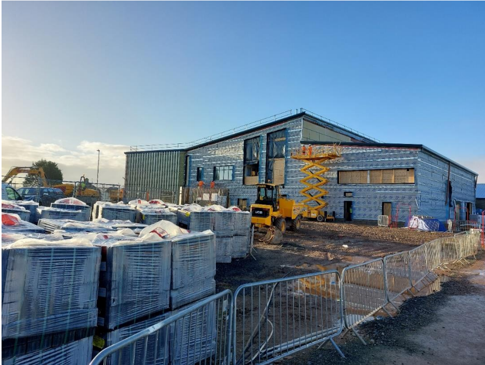
East elevation under construction
