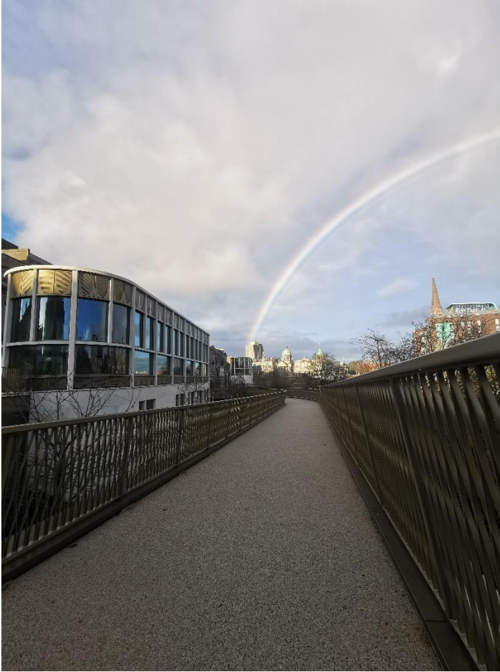
View from new ramp off Union Street
