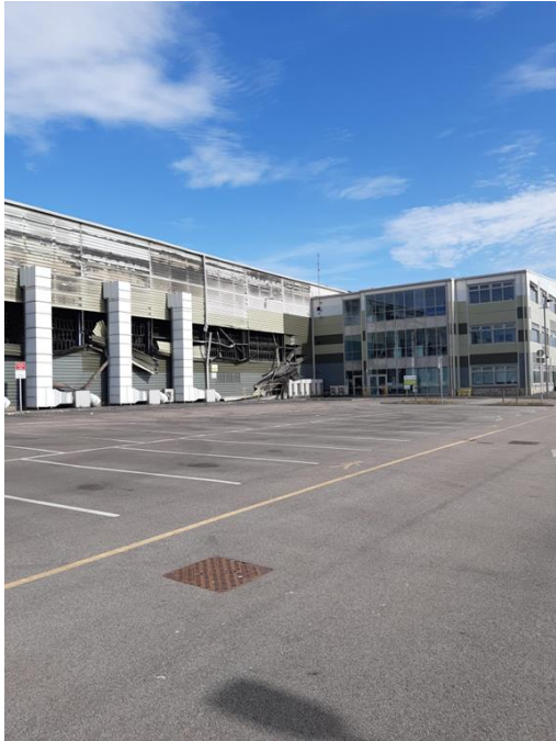
Post fire and pre-demolition.
