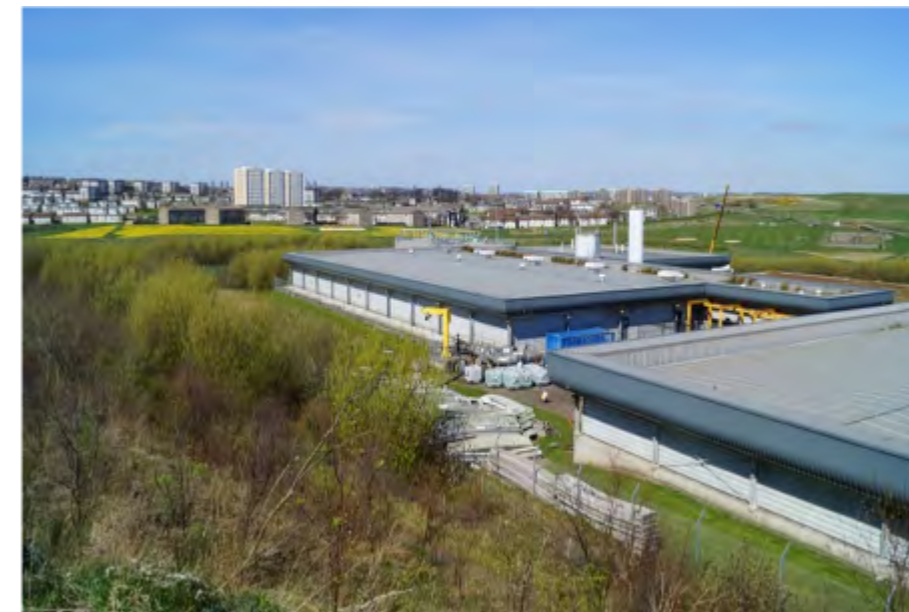
Nigg Waste Water Treatment Works
