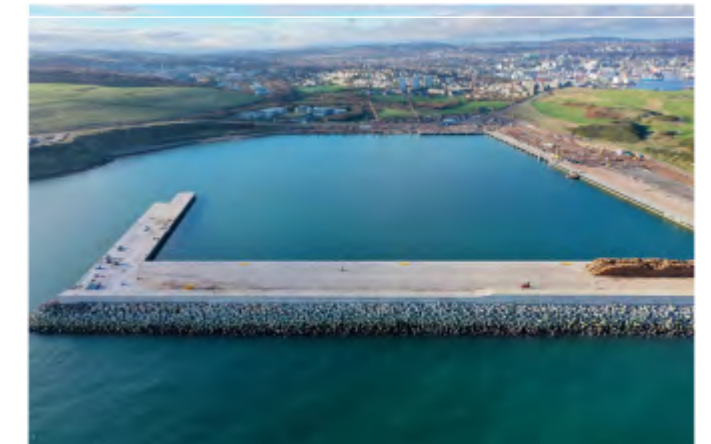
Development should be integrated with Aberdeen South Harbour and provide high-value activity that is a catalyst to further investment across ETZ.
