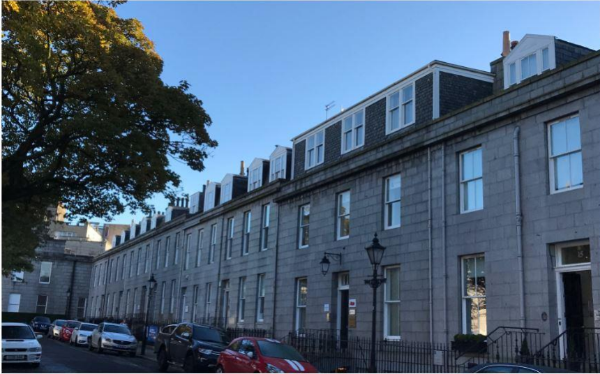
Example of a poorly designed roof extension – The modern box dormer is too large, thus it dominates the roof slope on an otherwise traditional terrace.
