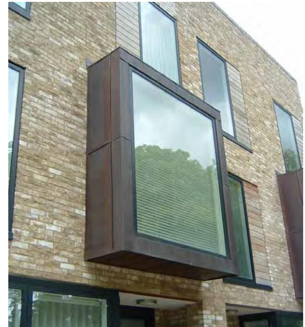
Accordia: pop-out windows providing special moment on elevation.
