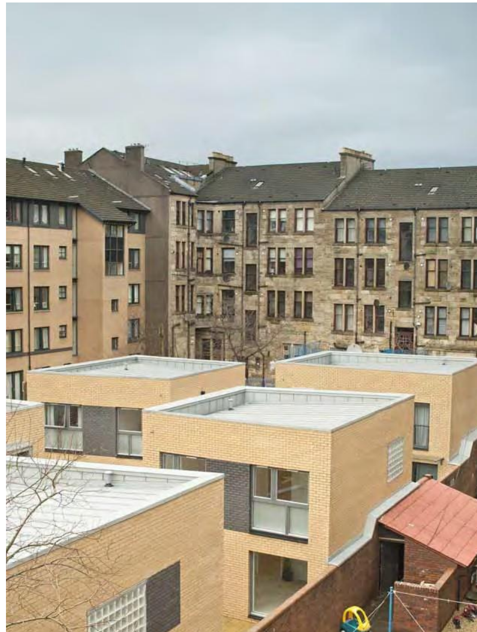
Fore Street: Flat roofs carefully considered alongside massing and proportions of buildings.
