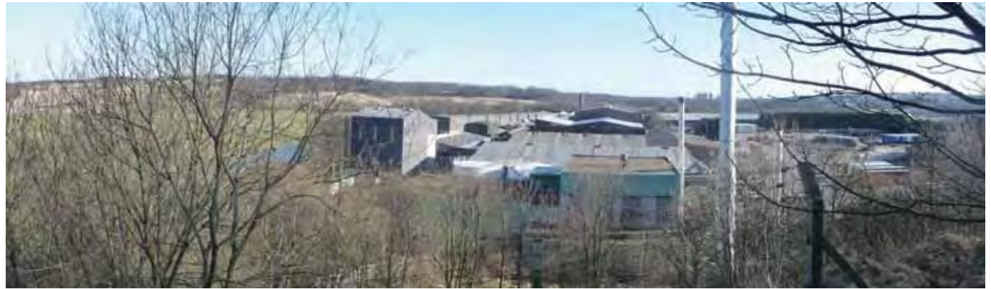
View east across the site from Danders Hill
