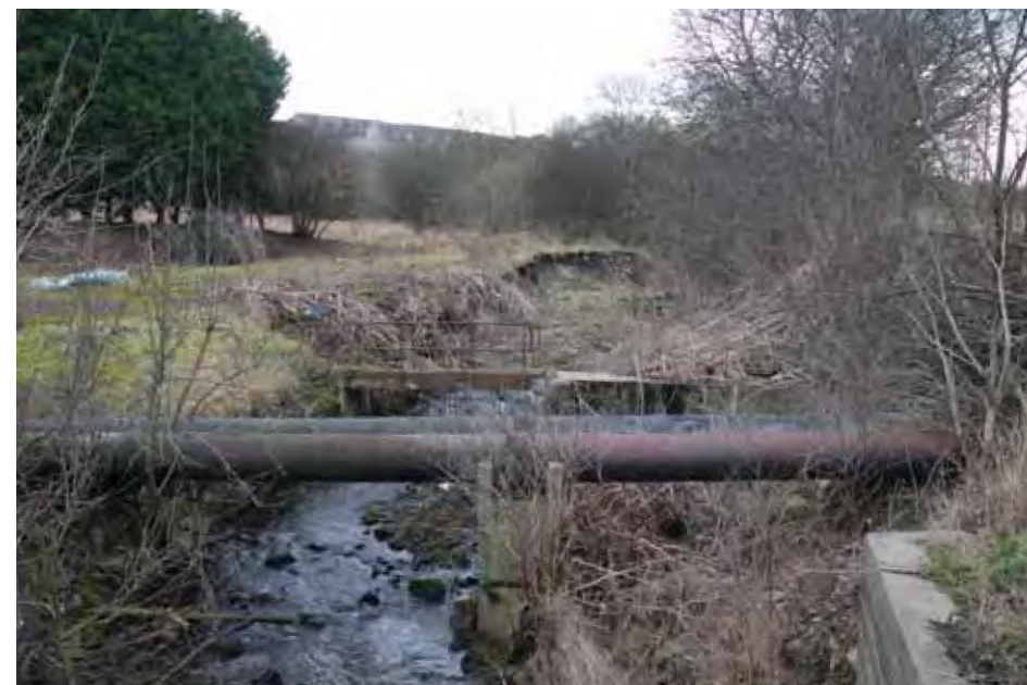
Remove redundant grilles, pipes and infrastructure
