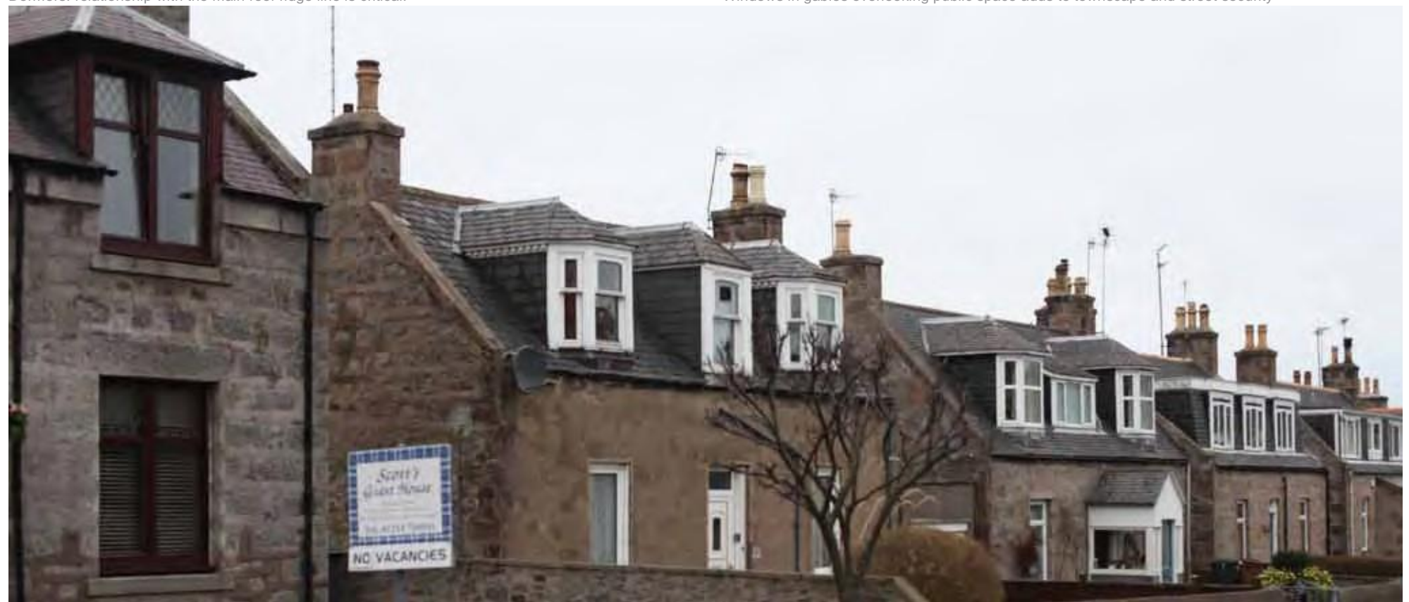
Dormers: position, proportion and size relative to the overall elevation should be considered.
