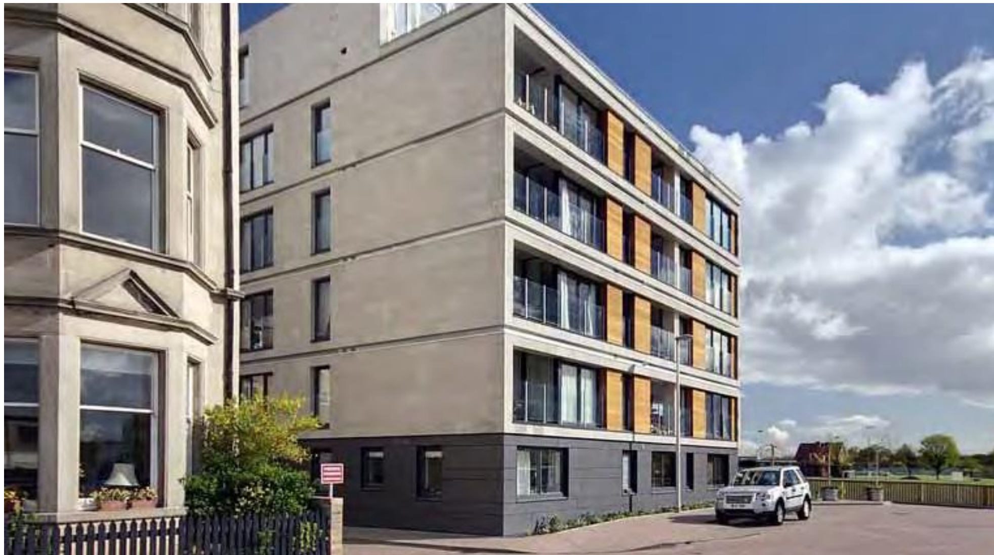
Bangholm Terrace, Edinburgh. Eternit cladding panels at ground floor. Untreated timber at balcony areas.
