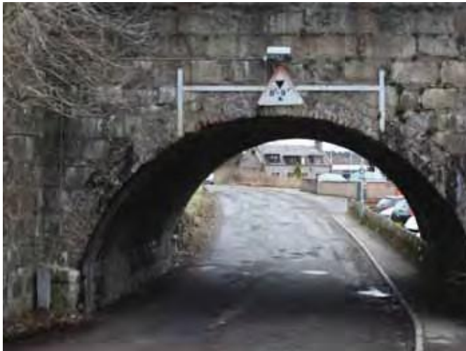
View 4: Rail Bridge at bottom of Station Road.
