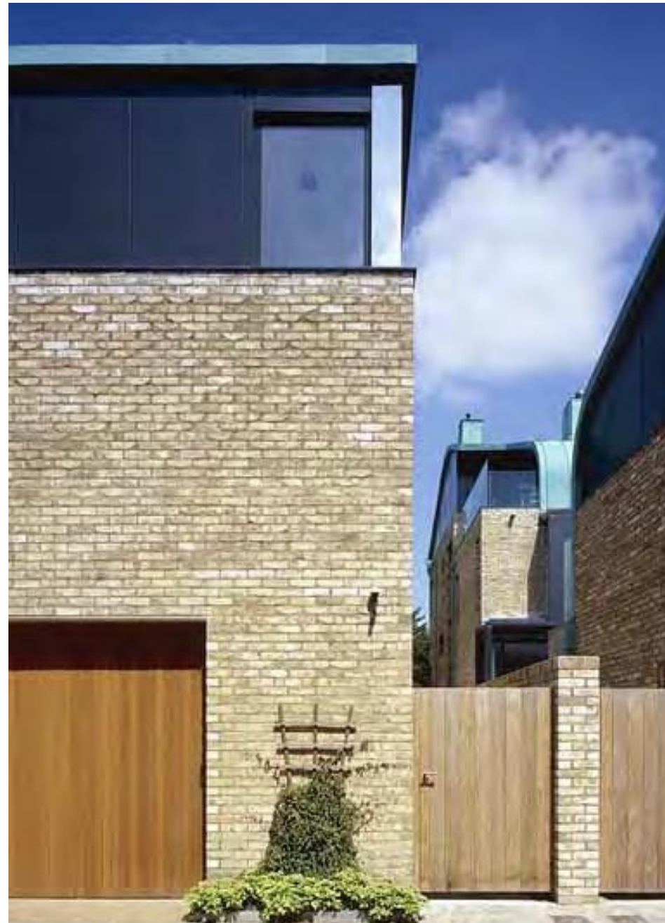
Accordia: street elevations carefully considered to provide vertical articulation.
