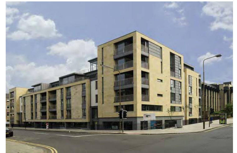
Eyre Place, Edinburgh. Eternit cladding panels at ground floor, top floor and accent areas.
