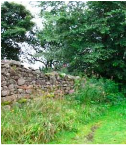
Figure 2.23 Existing stone walls on site
