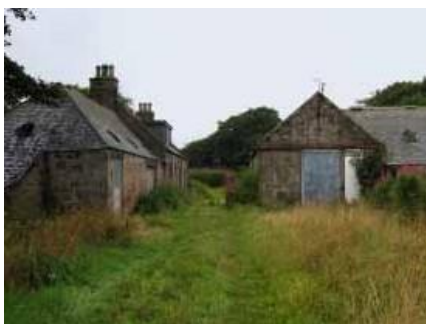
Figure 2.3 The existing farm buildings on site
