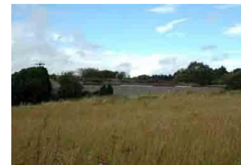
Viewpoint 17: Electricity Substation
