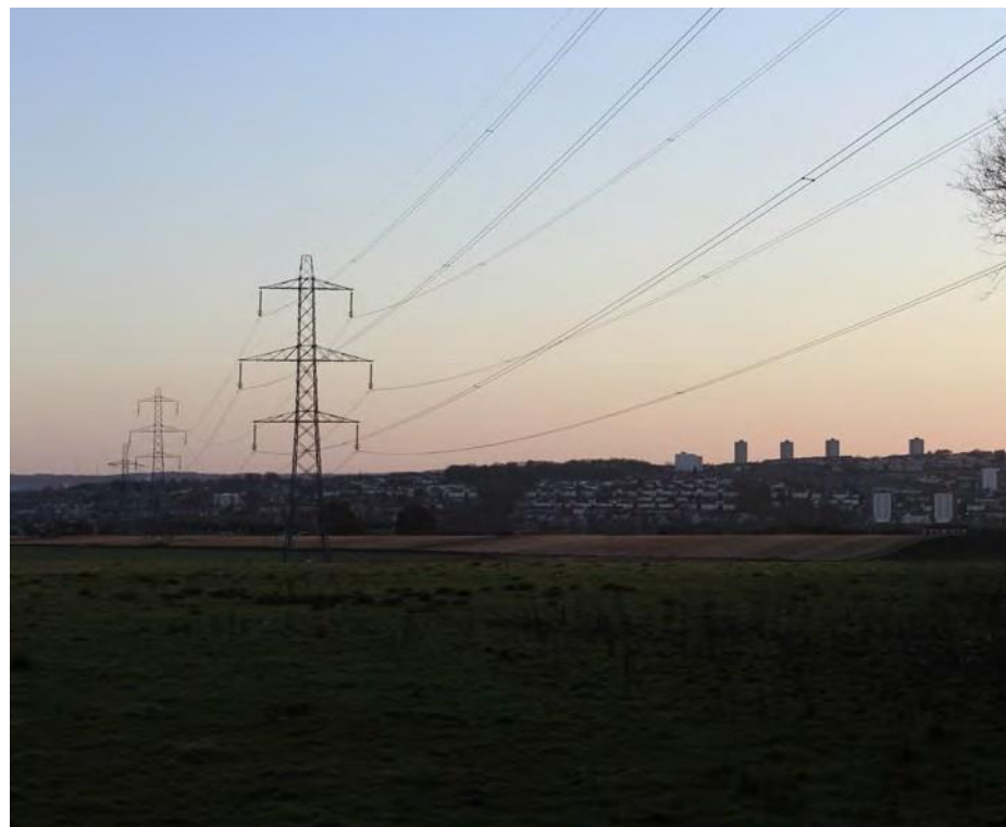
Figure 2.6: A row of pylons are a conspicuous feature in the south-east of the site
