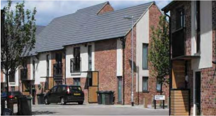
Two- and three-storey buildings addressing open space/entrance - Allerton Bywater
