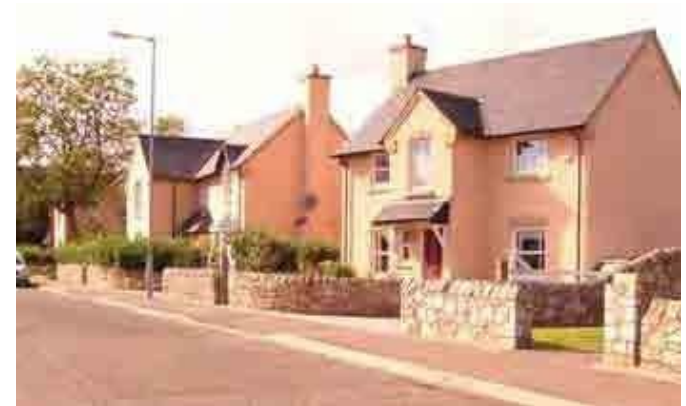
Well defined building line and plot boundaries, Scottish Borders.
