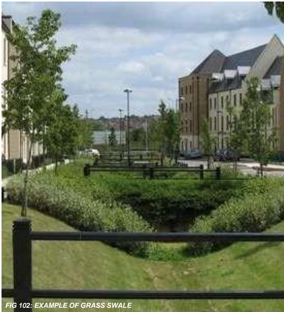
FIG 101: EXAMPLE OF GRASS SWALE
