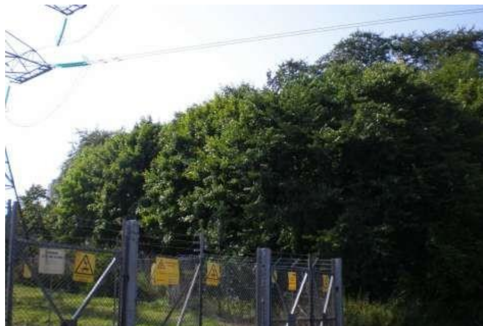
FIG 50: EXISTING SUB STATION COMPOUND
