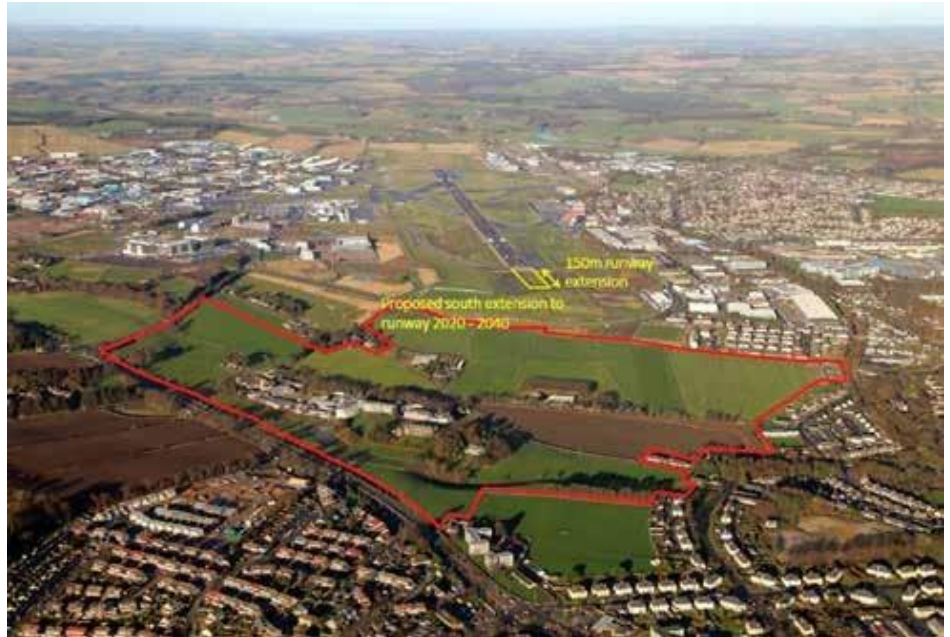
above Diagram Illustrating Proposed Runway Extension and it's Relationship to the Site
