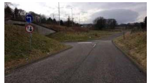
above Approach to Underpass
