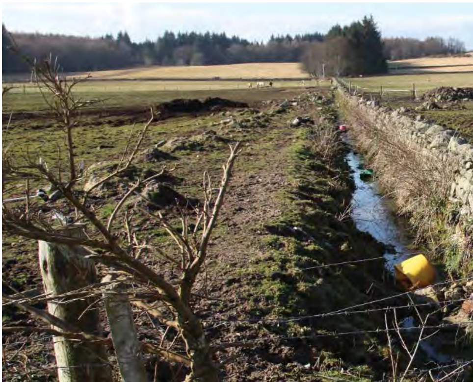
fig. 37: Existing field drainage ditches
