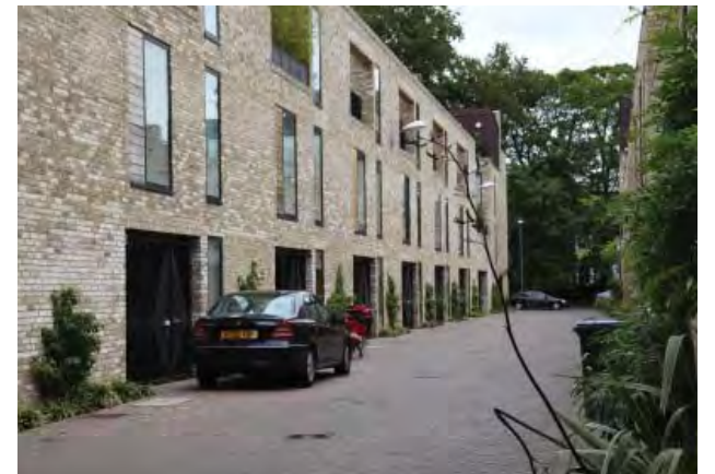
fig. 88: Residential street - Accordia, Cambridge
