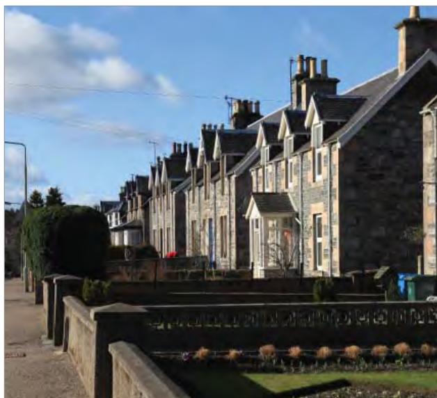
fig. 168: Residential frontage to street, Granttown on Spey
