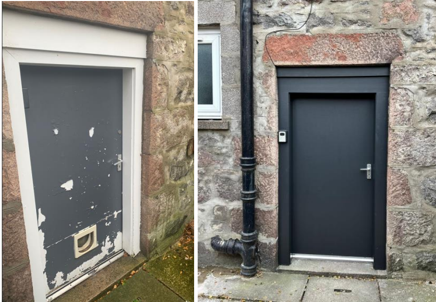
Figure 9 & 10 – Renovation of rear property access to garden area
