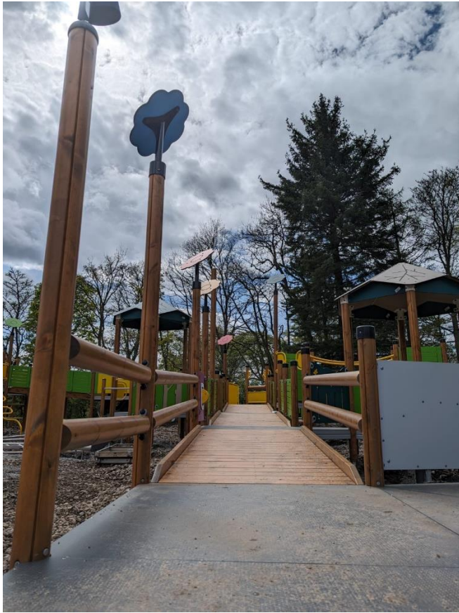
Accessible unit – wide access to allow those of all abilities to take part in play.
