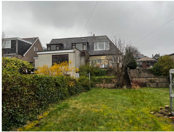
Rear view of appeal site, existing small garden room extension. Adjoining property at 23 Balgownie Crescent includes large rear extension and side extension.
