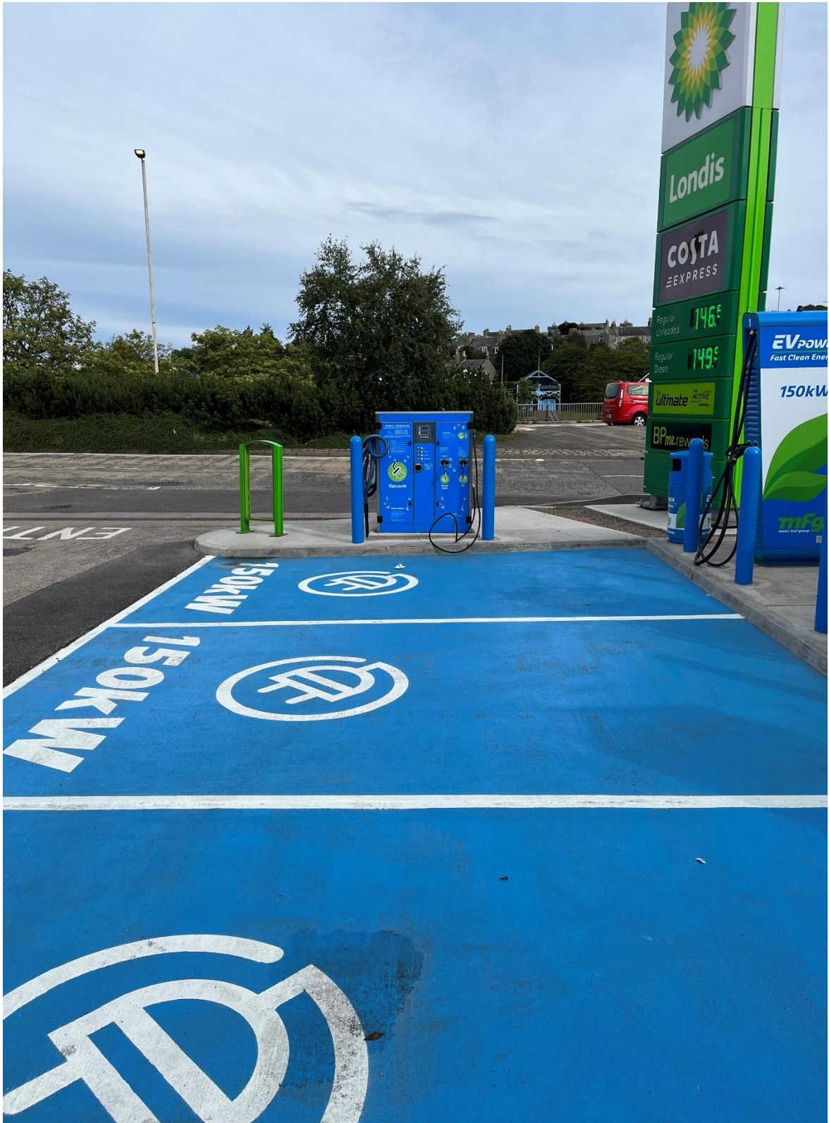
The Additional EV charging bays can easily be used as temporary parking bays for none electric vehicles
