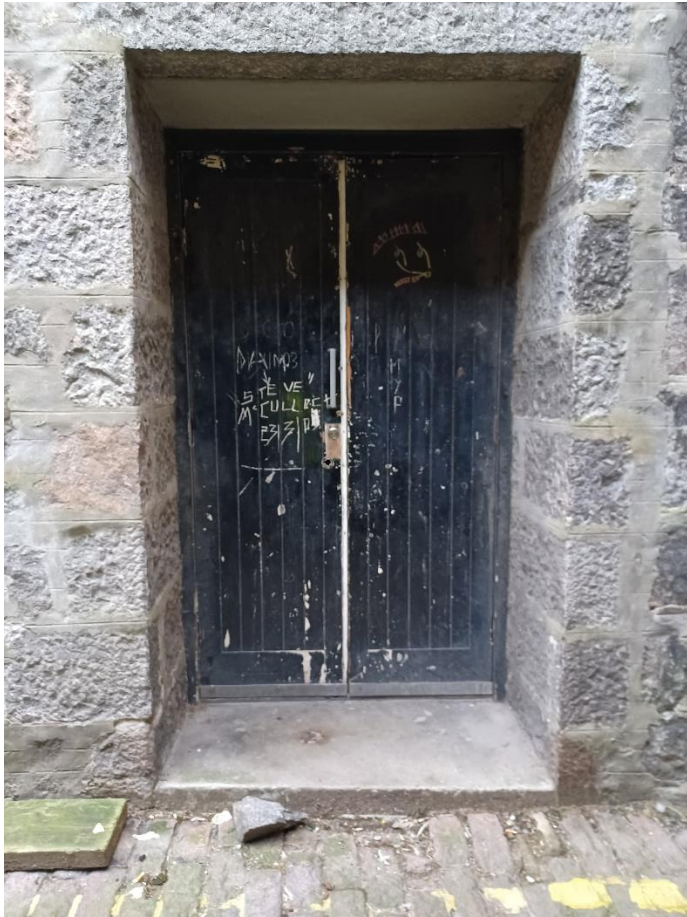
1. Basement door to be replaced
