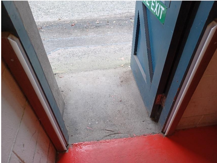
2. Door 2 – existing internal flood barrier mountings
