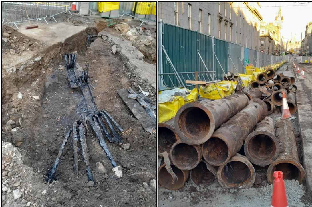
Removal of redundance cables & pipes
