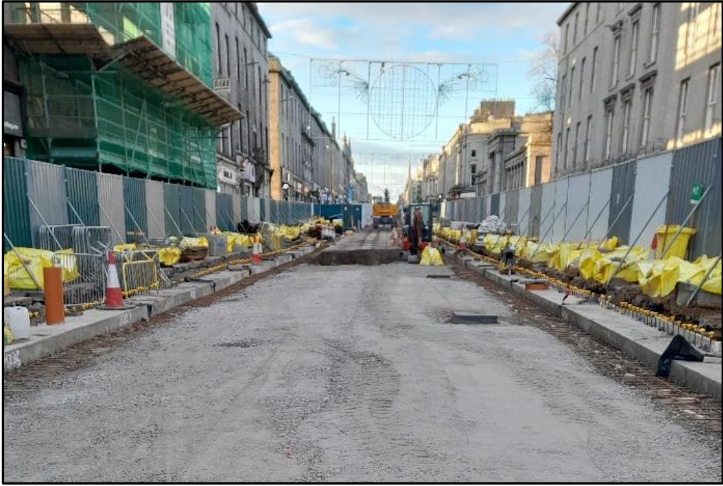
Kerb Log & Preparation of Sub-base
