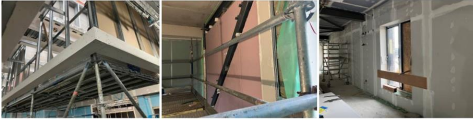
Sheeting to roof lights, Fireline to Stair 1 and 1 st Floor sheeting
