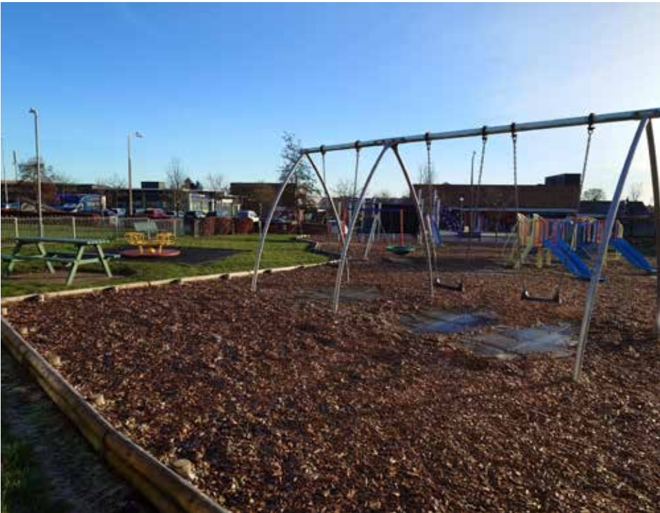
Figure 112: Image of raised edging and loose surfacing at Greenfern Road Play Area
