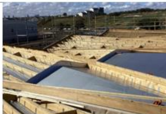
Photo 3- C1 Amphitheatre warm/cold roof details
