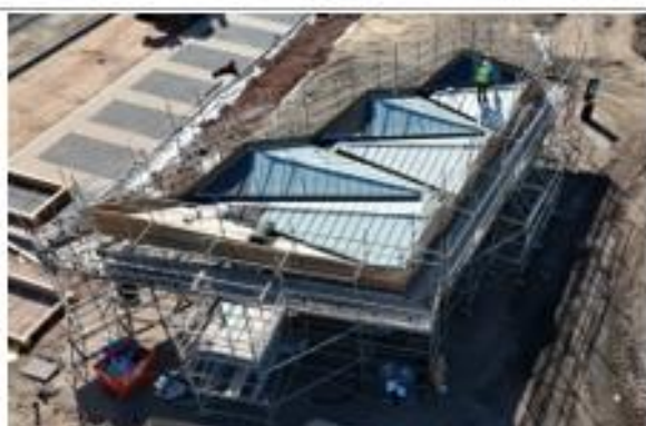
Photo 2 – Canopy roof and gutters complete
