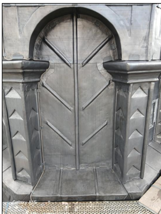
Completed leadwork to roof
