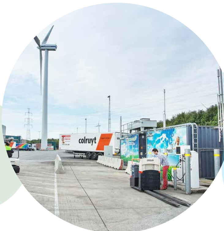
Hydrogen refuelling station at the logistic centre of Belgian retailer Colruyt. Hydrogen is produced via electrolysis using renewable wind energy. This station has been operational since February 2012.
