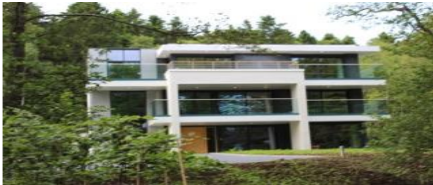
Plot 4 as completed - 46/48 Culter House Road
