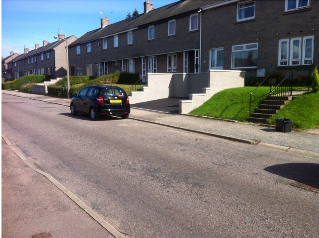
Driveway and retaining walls.
