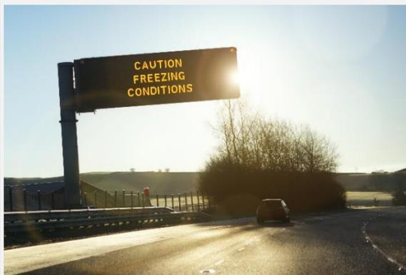
Figure 4-16: Cantilever VMS sign
