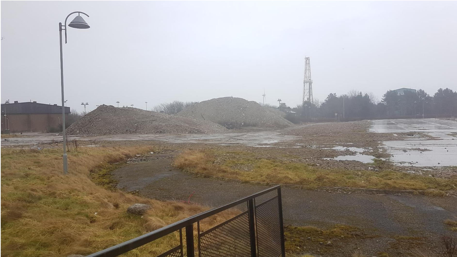
LOOKING EAST ACROSS INTERIOR OF SITE
