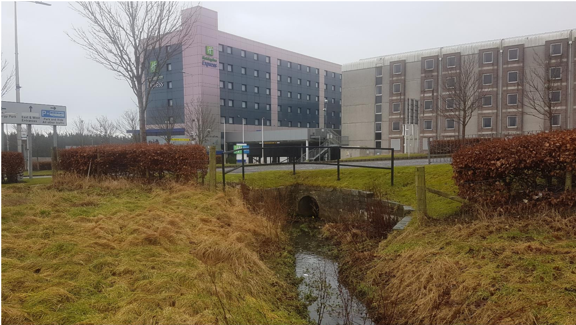
LOOKING SOUTH: CULVERT UNDER PARKWAY EAST
