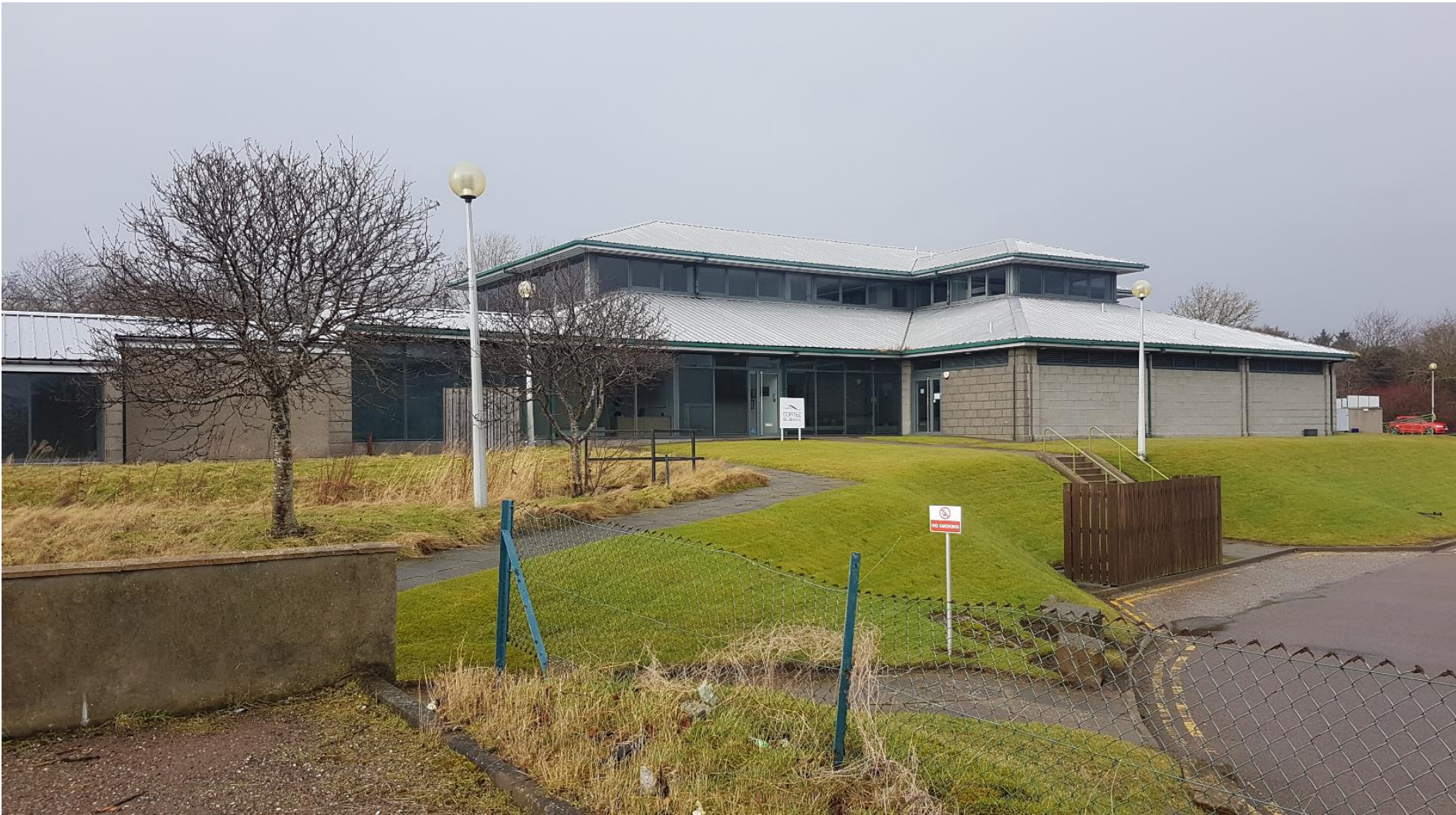
SILVERBURN LODGE, ADJOINING NW CORNER OF SITE
