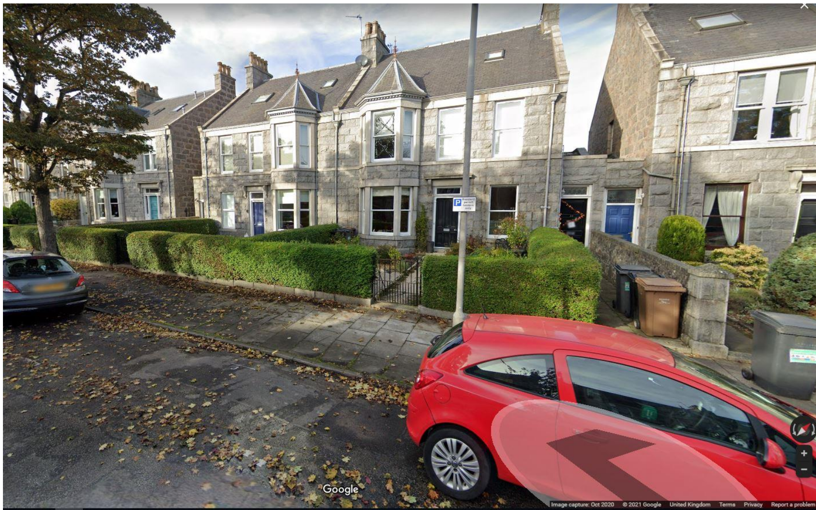
Google Streetview Image October 2020 – Prior to the disabled bay installation
