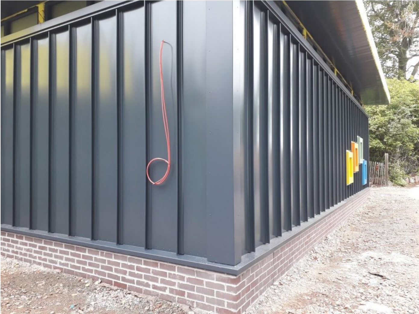
Duthie Park – East Lodge Extension Progress Photograph
