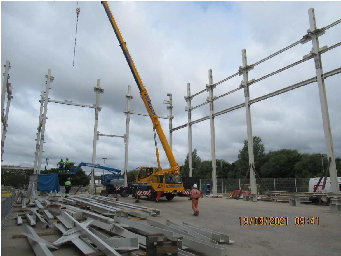
Waste Reception Hall Steel Structure Installation
