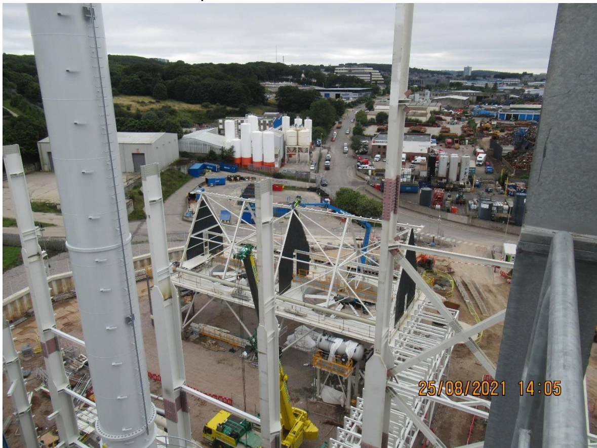
View West from Boiler Superstructure
