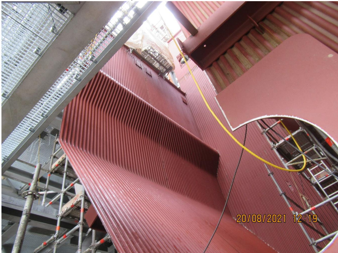
Boiler Construction Underway
