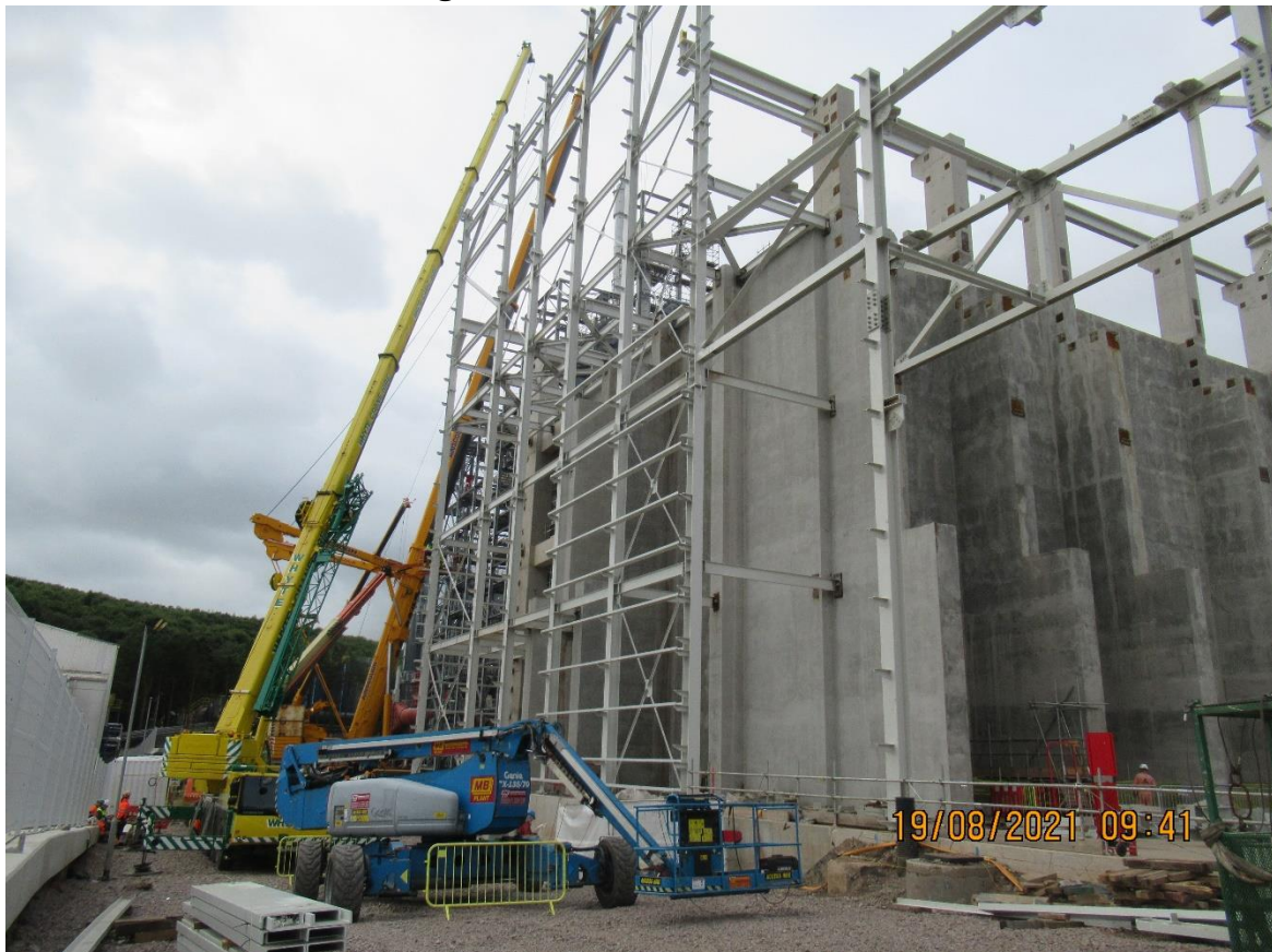
Waste Bunker and Building Steel Structure
